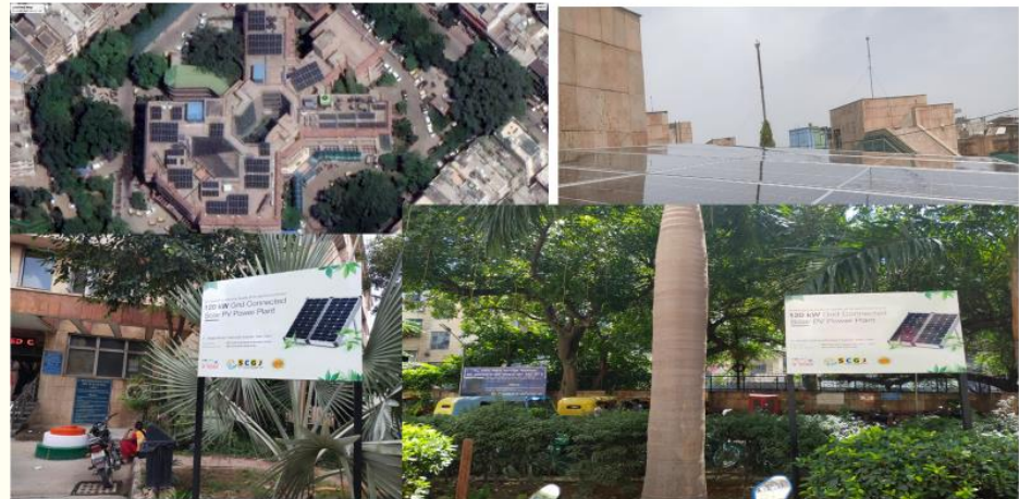
Solar Project at Madan Mohan Malviya Hospital
