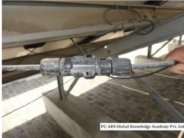
Fig. 8.5.4 MC4 connector
