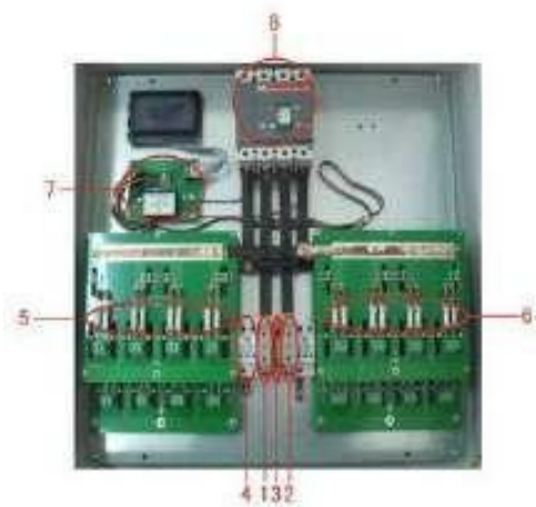
Fig. 8.3.4 A typical combiner box connection area
