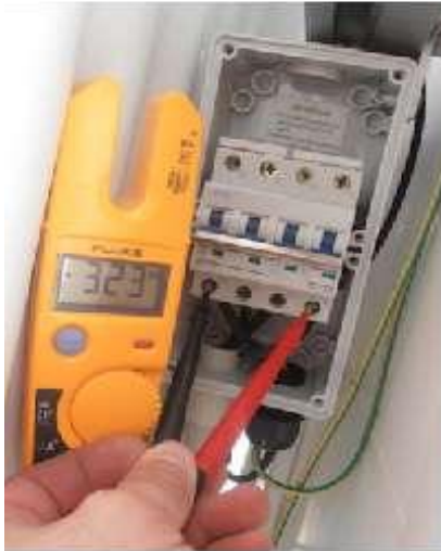
Fig. 9.3.5 Checking of reverse polarity using a clamp-on meter (Voltmeter)
