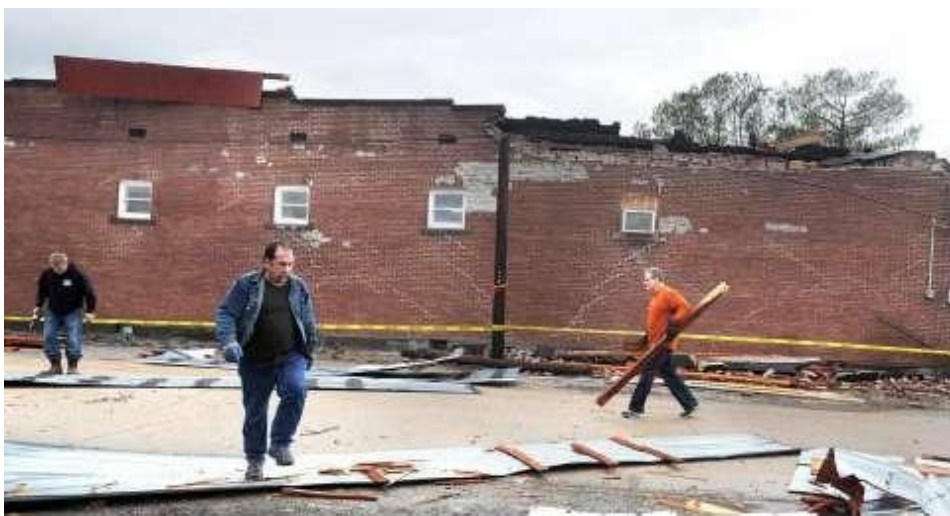
Fig. 8.1.1 Clear site area before installation
