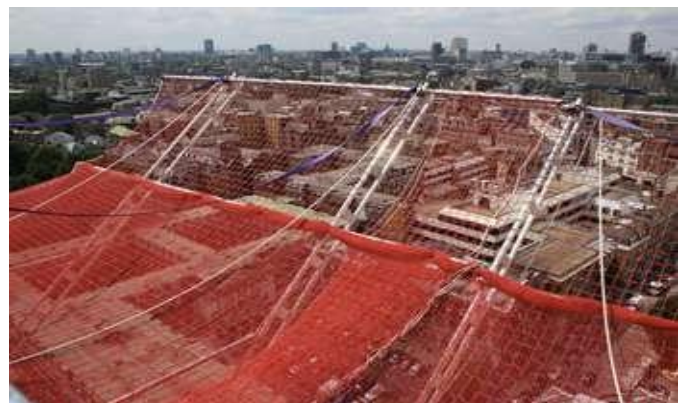
Fig. 11.4.6 Safety Nets for High-Rise buildings
