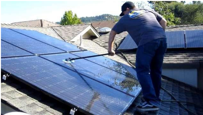
Fig. 10.2.2 Cleaning modules using a mop
