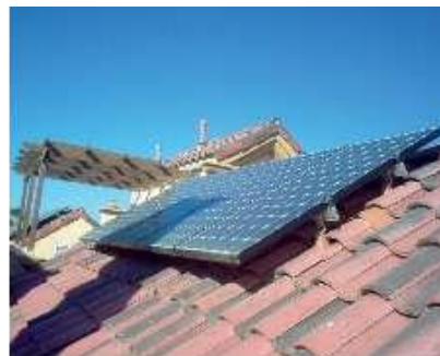
Fig. 9.3.1 Spot shading causes hot spot and may damage a module
