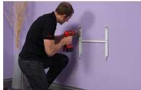
Fig. 8.2.6 Installation of Inverter mounting structure
