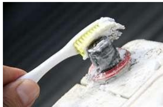
Fig. 10.2.11 Cleaning of batteries terminals to avoid corrosion and loose connections
