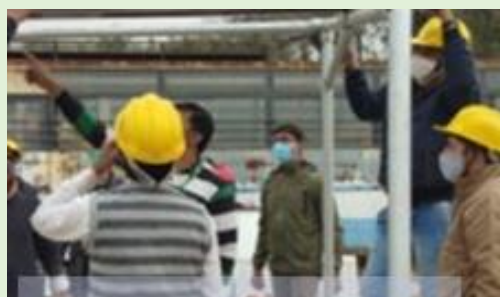
Solar Power Plant Installation
